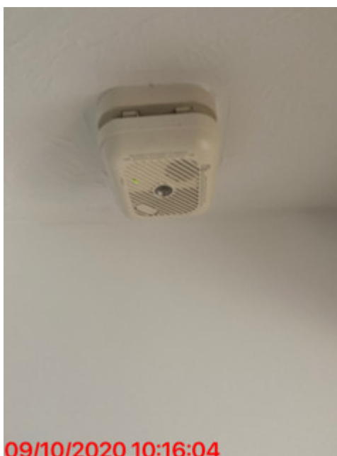
Smoke alarm at bottom of stairs
