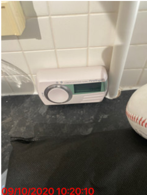
Kitchen carbon monoxide alarm
